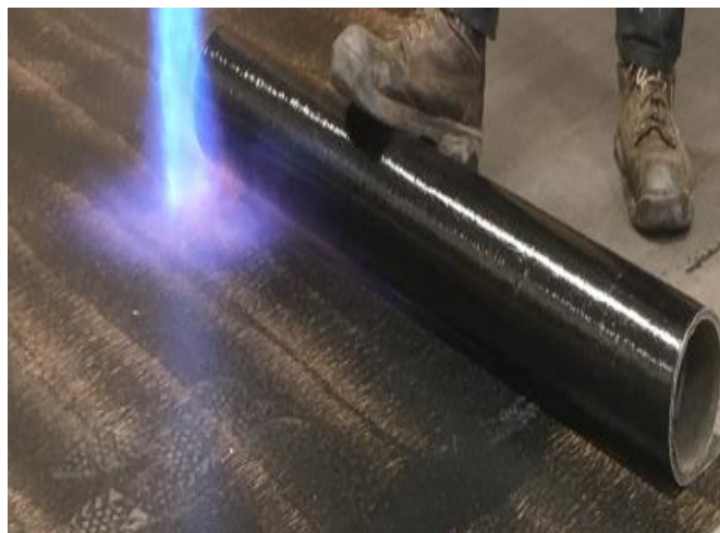
Figure 3 - Typical torch on method of application
